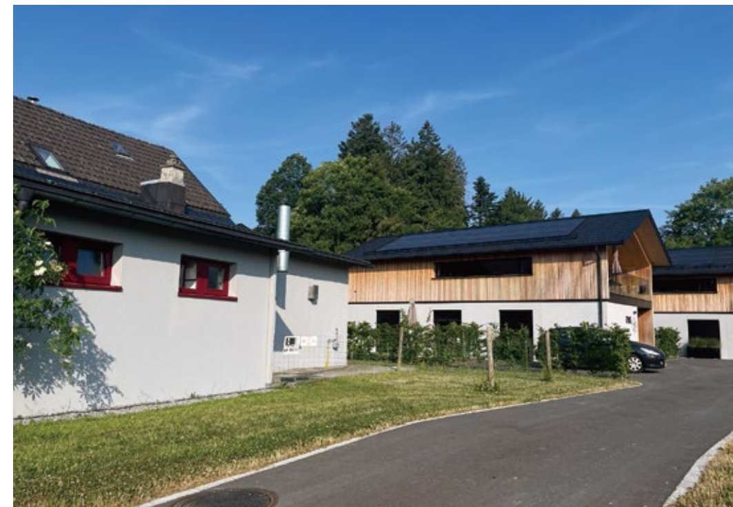
02 Residential ESS Project in Europe
