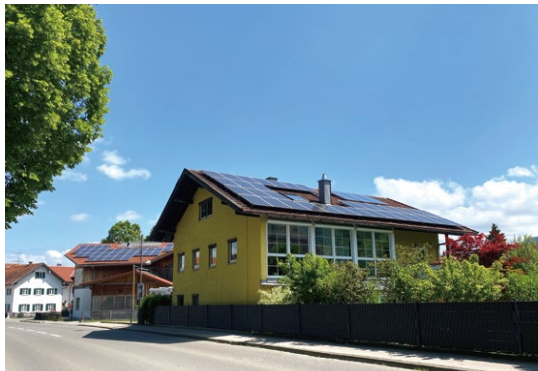
01 Residential ESS Project in Europe
